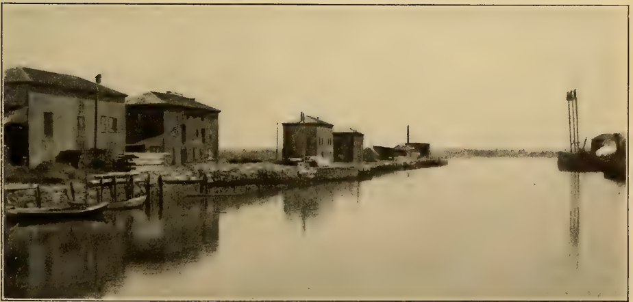
Derby Wharf where the East India ships once lay three deep. These decaying warehouses were filled with the riches of the most remote lands a century ago.
